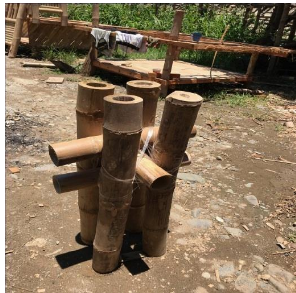
Fig. 4. Column and Beam Connection.
