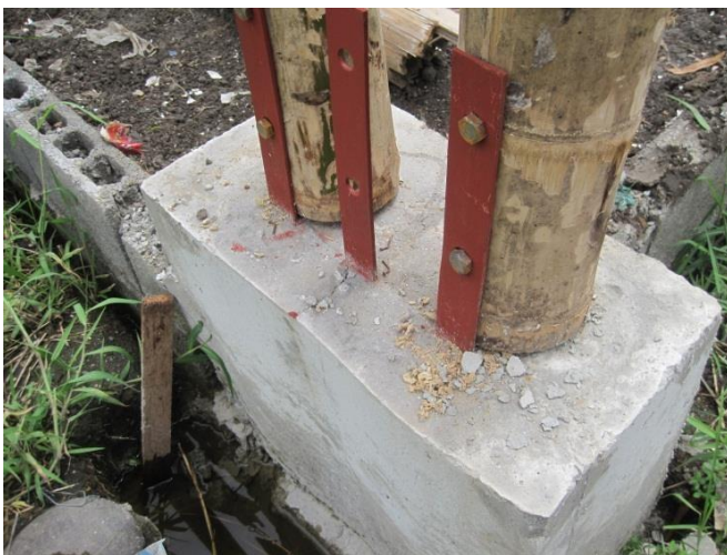
Fig. 6. Column and Foundation Connection.
